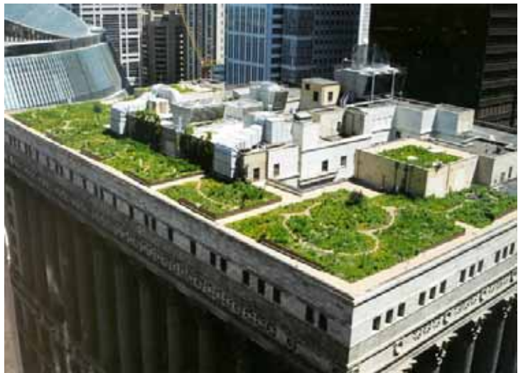
Figure 6.2 The city hall after installation of the green roof in summer 2004 (City of Chicago).
